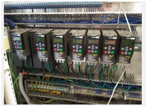
PLC-VFD Automation Panel
